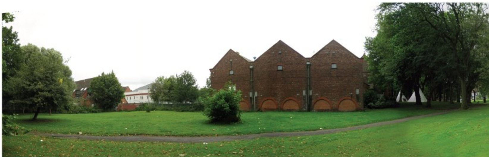
The west of the building is blank and has no contact with the park - it is very much a rear. Consequently this area of the park feels neglected.
